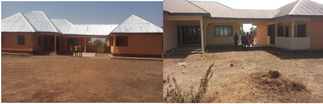
Uncommission Completed CHPS Compound at Nagbai and Gadantinga
